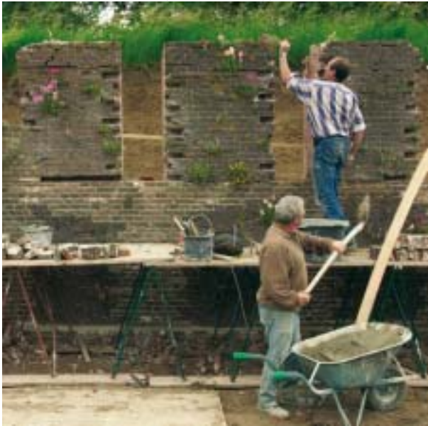
Plant conservation, Gorinchem fortification wall, photo: Marcel Köppen
