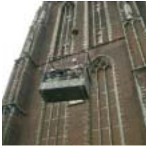
Survey of the Sint Jan tower
