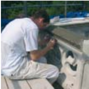
Restoration of balustrade
