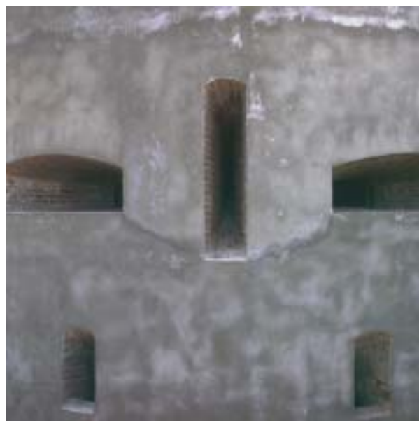
Capponière Gorinchem fortification wall, photo: Marcel Köppen
