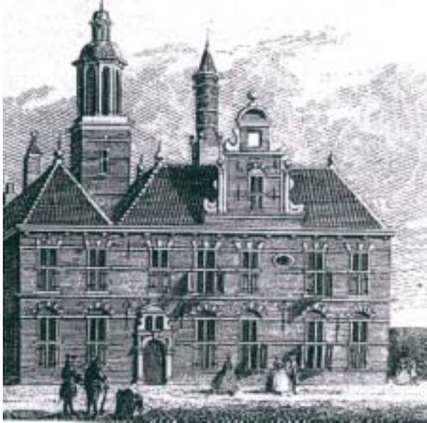
Condition before restoration
