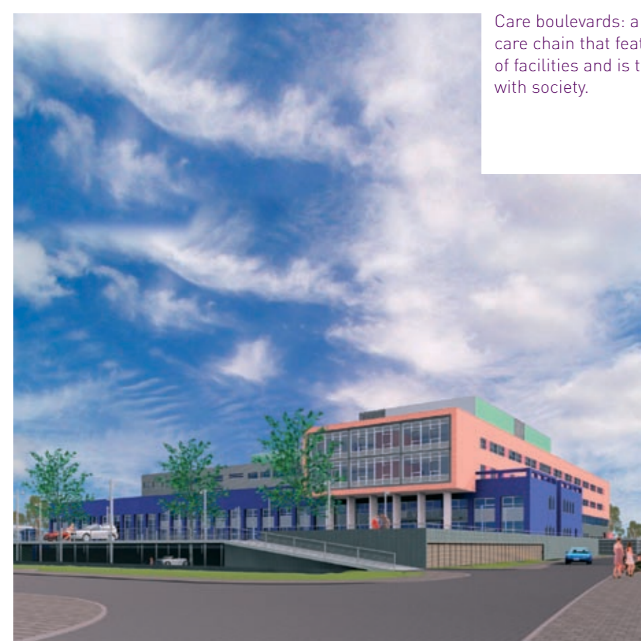
Northern view of Rijnland Hospital
